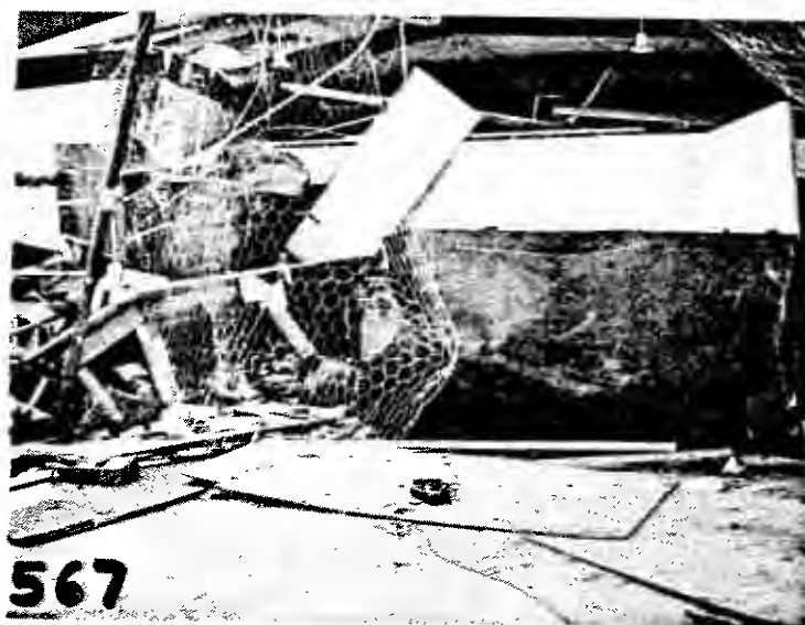
FIGURE 17. VIEW OF TANK NO. 3 INSIDE STRUCTURE 24
