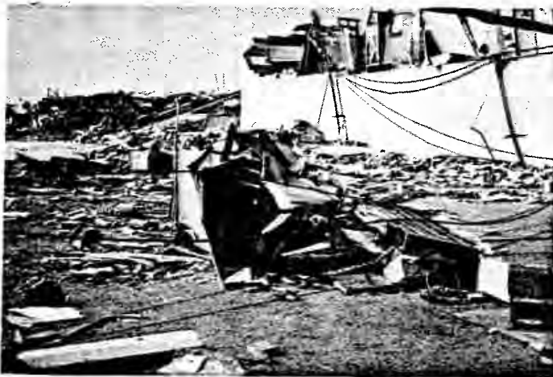
FIGURE 6. VIEW OF DESTROYED COMPRESSOR NO. 1
