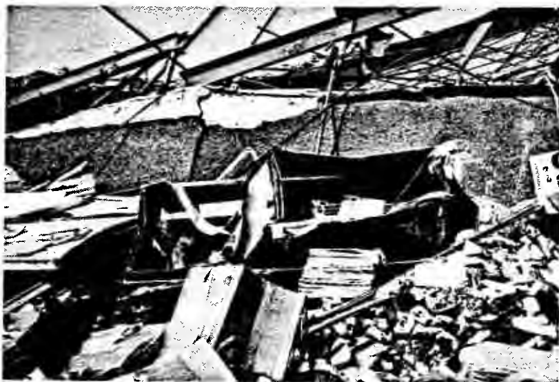
FIGURE 7. VIEW OF DESTROYED COMPRESSOR NO. 2
