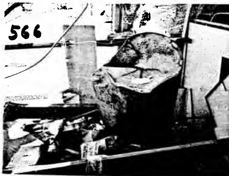
FIGURE 16. VIEW OF TANK NO. 2 INSIDE STRUCTURE 24
